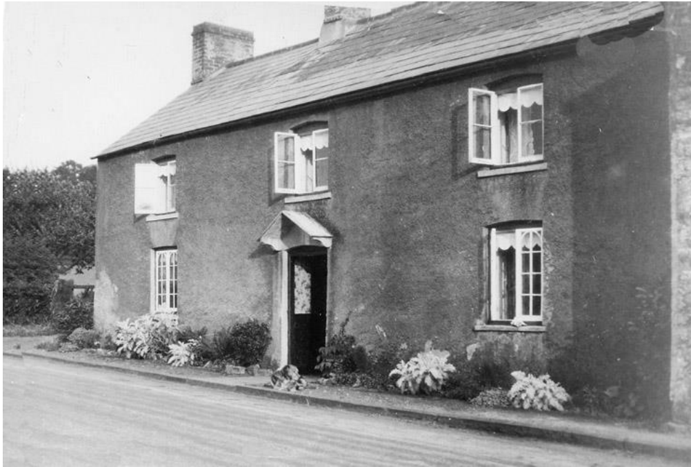
The Laurels, this house was demolished circa 1968.
